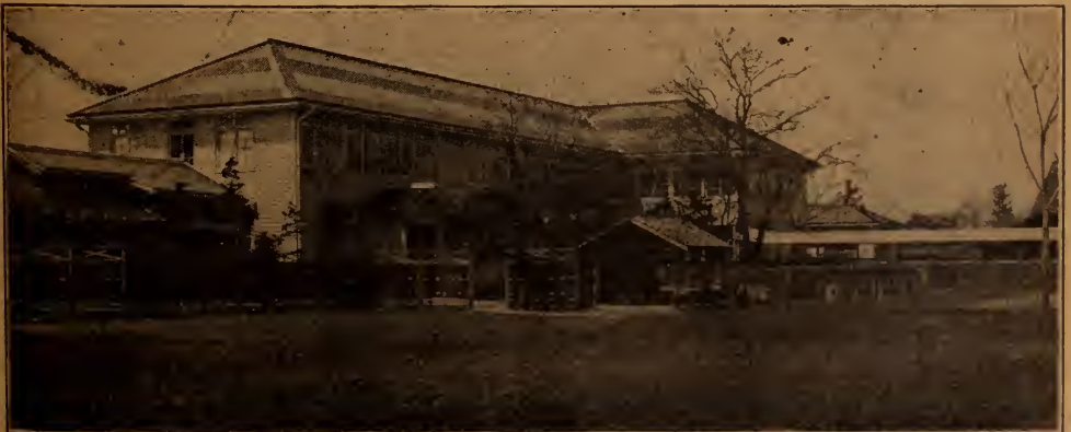
DORMITORY, NORTH JAPAN COLLEGE, ERECTED IN 1906.
